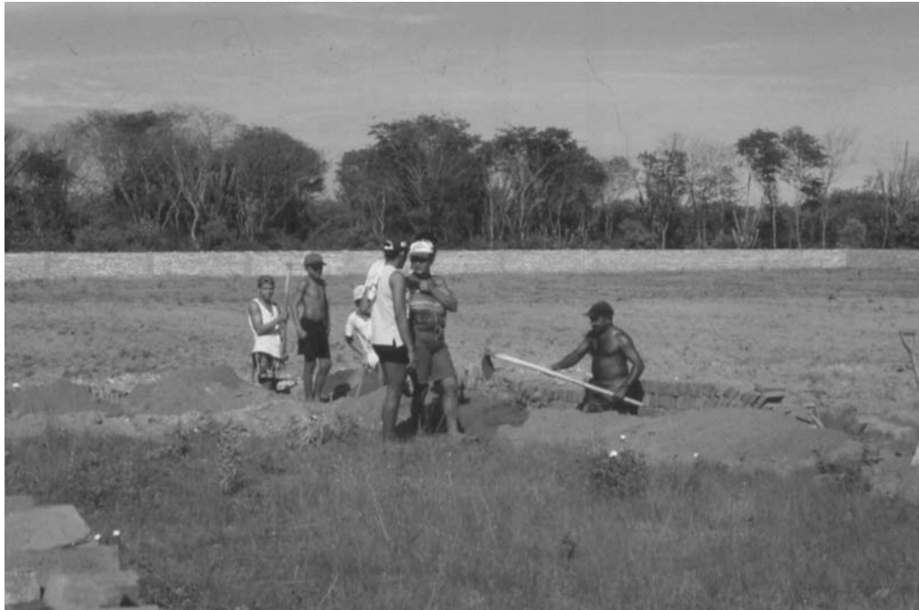
FIGURE 6. Chapel construction as part of the cash-for-work program.
