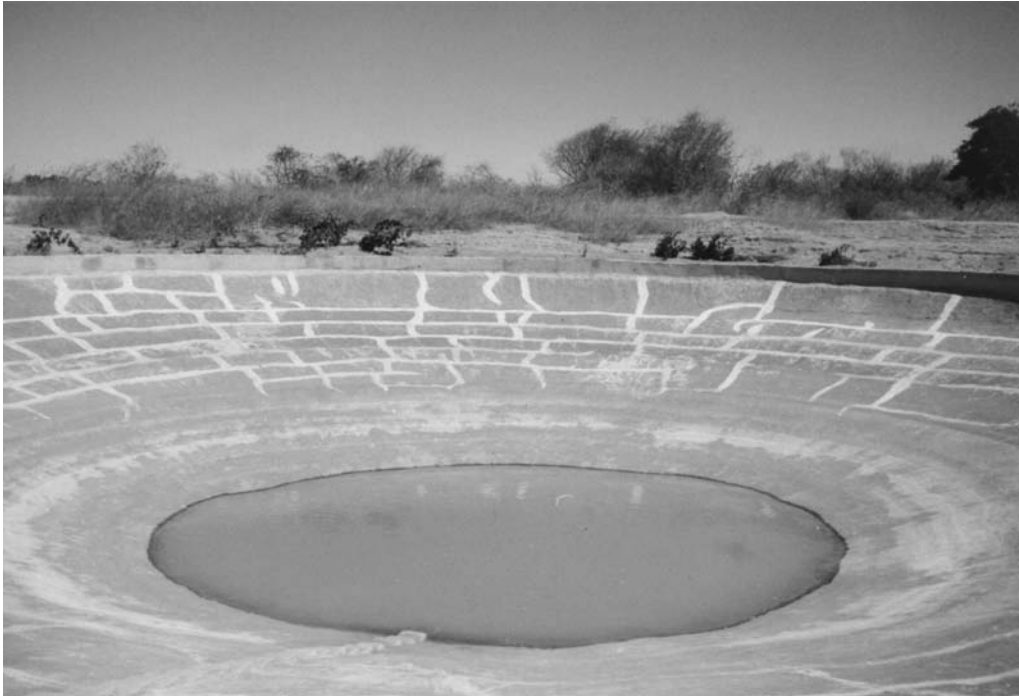
FIGURE 4. A barreira (water-runoff catchment system used for domestic and livestock needs).
